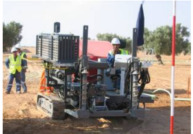
← The pilot bore begin.
