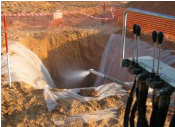
→ During the pilot bore the bentonite transports the sand backwards.
