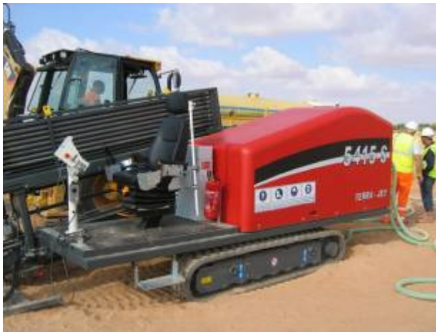
← The TERRA-JET 5415 S is ready for the pilot bore.
