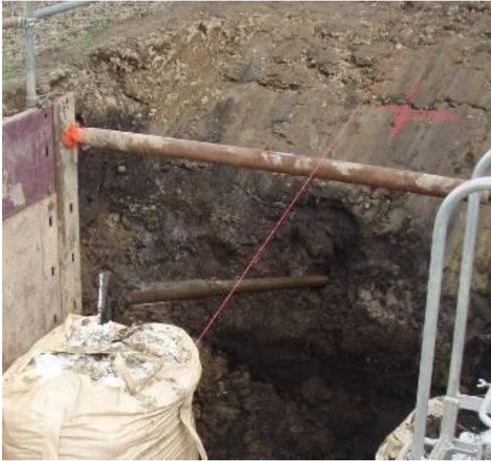
The drill head reaches the target pit.
