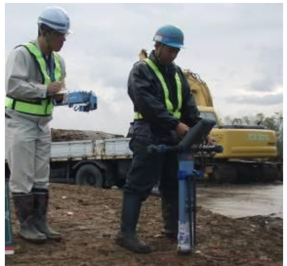
The pilot bore is located and documented.
