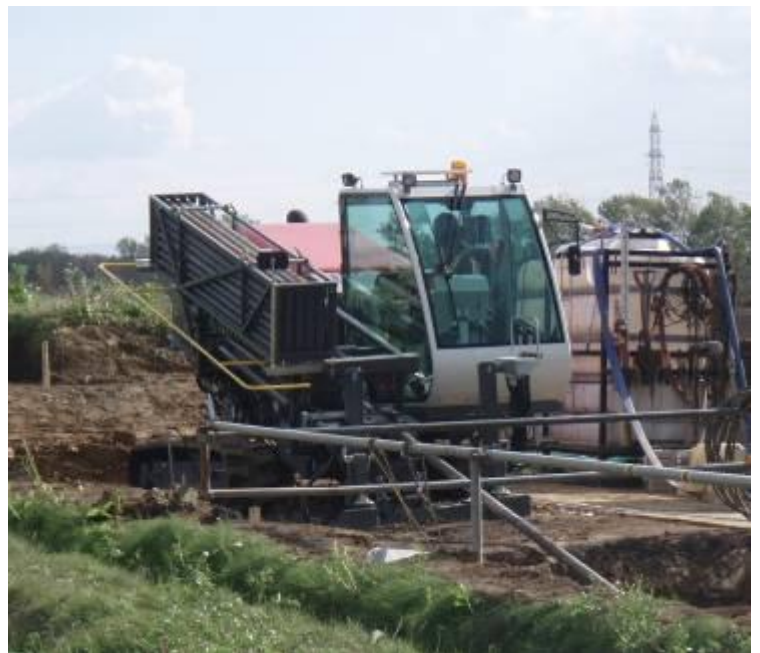
The TERRA-JET 8522 S after the successful pipe pulling.
